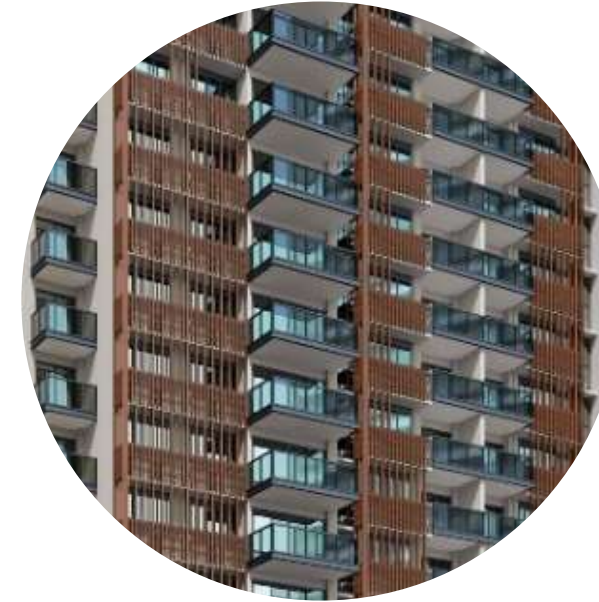
Signature Tower Façade Screen
